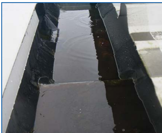
Typical sump unit serving a side box outlet
