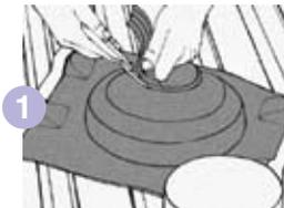
1 Trim the cone to suit pipe size, using a sharp pair of tin snips. Not a knife.
