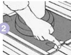
2 Lubricate the pipe with water, slide the soaker flashing down the pipe and form to suit the roof profile.
