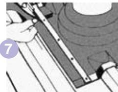
7 Fasten side strips provided and trim excess soaker where necessary. **Note:** Side trimming of the soaker should be determined prior to cutting roof.
